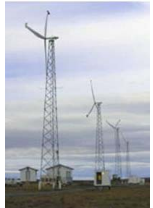
Remote & Wind-Diesel (50 – 300 kW)
