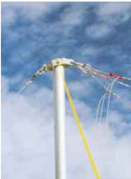
Above: The gin pole bracket showing the hoisting cable (left), nylon rope for steadying, and three lifting guys to tower (right).
