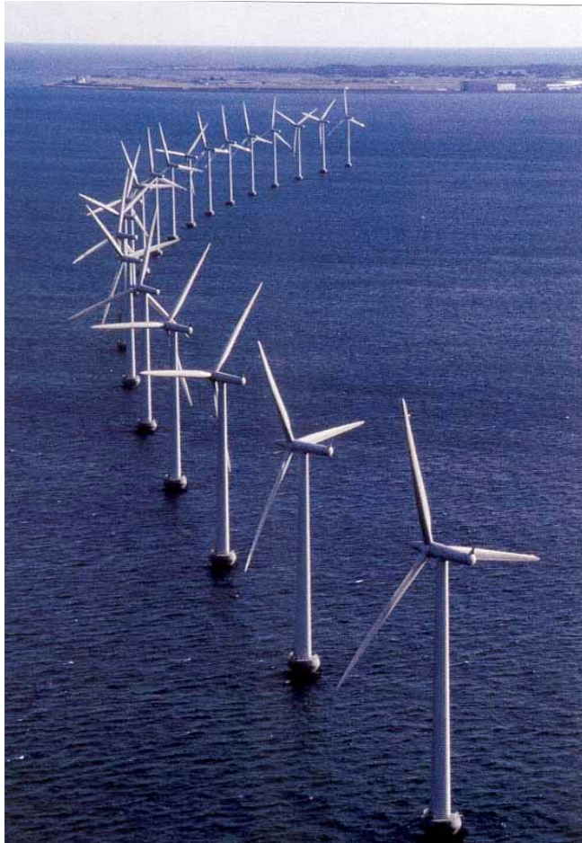
Middelgrunden: The latest and largest wind power co-operative in Denmark, just off the coast of Copenhagen. More than seven thousand members own this 40 MW offshore wind park together with local utilities. It was inaugurated in May 2001.
