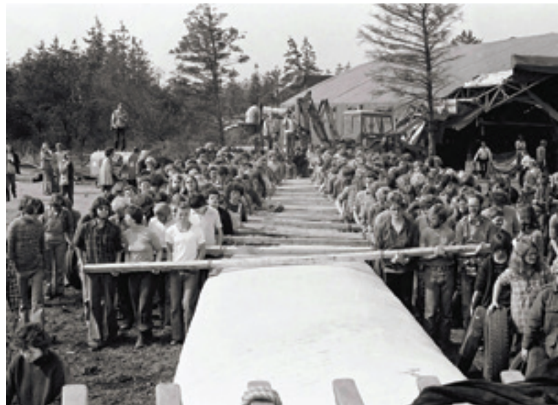
Figure 4-12. Tvind people power. The photo seen around the world in 1978 as students at the Tvind School carry one of the wind turbine blades from its assembly hall to the wind turbine. The action sent a political message: Together we are strong. We want wind power and we will build it ourselves. (Tvind School)
