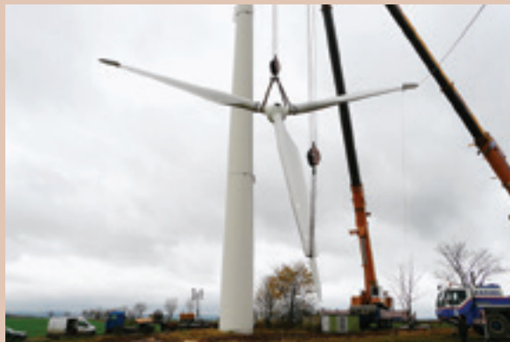
Lowering the rotor to the ground for disassembly.
