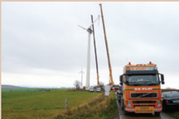
Removing the rotor from the nacelle.
